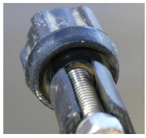
It is important that the nut is tightened in such a way that the collar is held in the groove in the nut.
